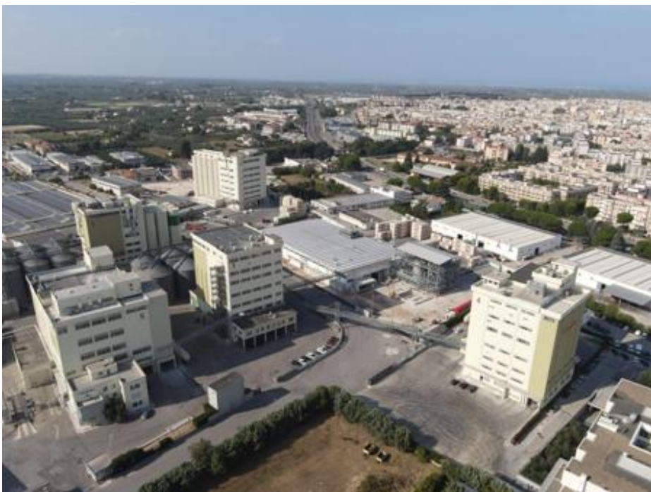
Figure 2 The five milling plants and the Casillo Next Gen Food plant seen from above
